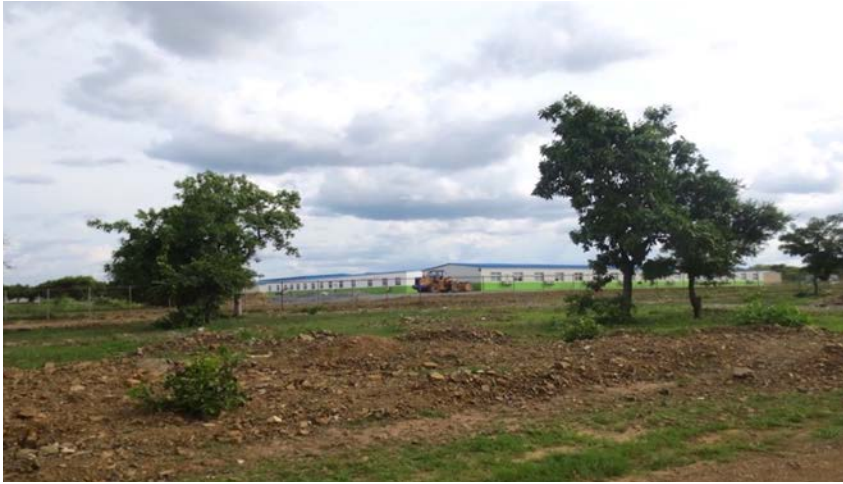
Shaanxi Mining Company's living quarters and offices for the Chinese workers at Gbane
