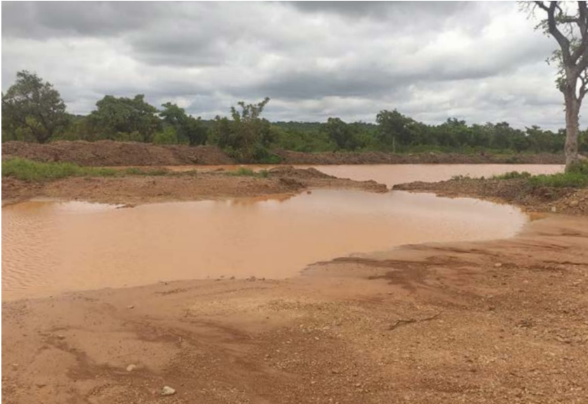
Sinkholes created by mining companies as a result of construction of a road to the mines
